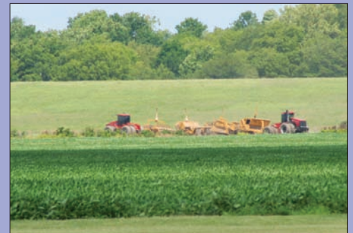
Landforming near the Toe of the Levee
