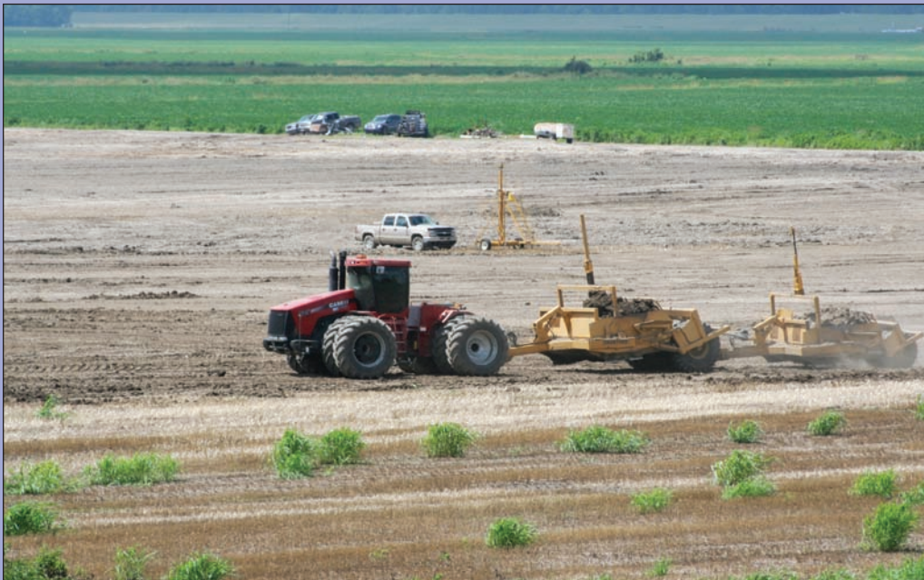
Landforming near the Toe of the Levee
