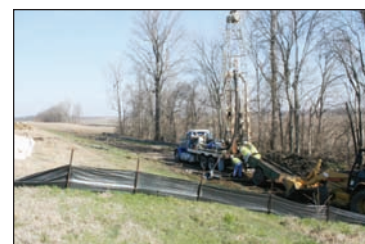
Francis – Installing Relief Wells
