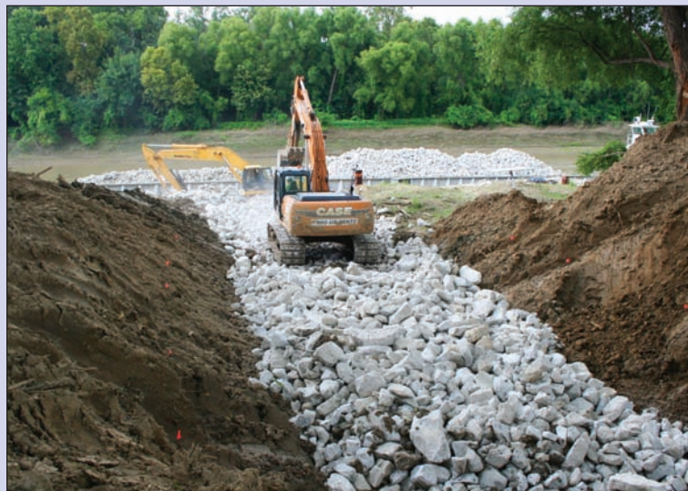
Yazoo River – Placing Rip Rap Rock in Tie-Backs
