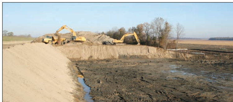
Francis – Berm Repair
