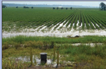
Francis Relief Well Flowing, Seepwater in Field & Irrigating
