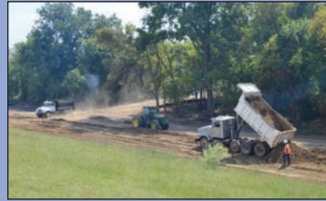
511L - Dumping material for base enlargement
