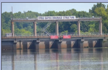
Steele Bayou Drainage Structure
