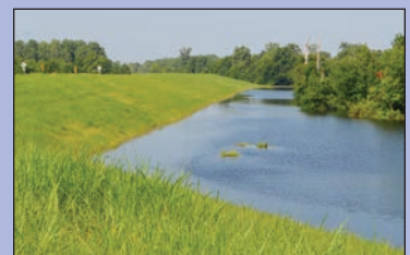
Water against the Levee
