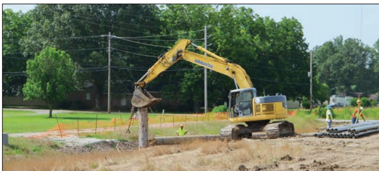
AVON - Pushing down Surface Casing
