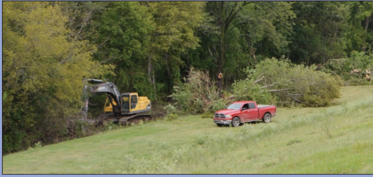
511L - Clearing the riverside toe
