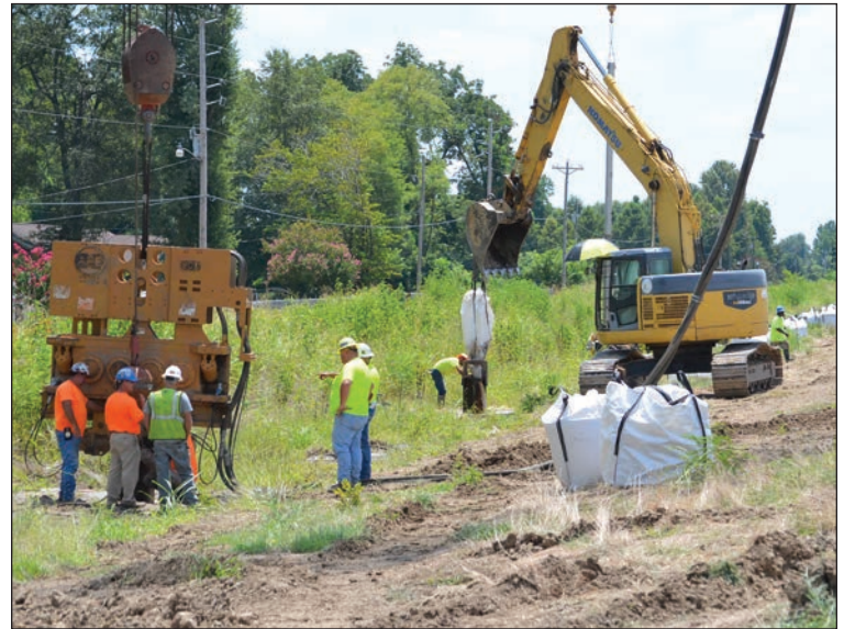
AVON - Placing Sand Filter Pack
