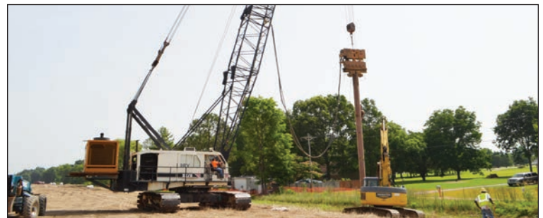
AVON - Vibrating in the Well Casing
