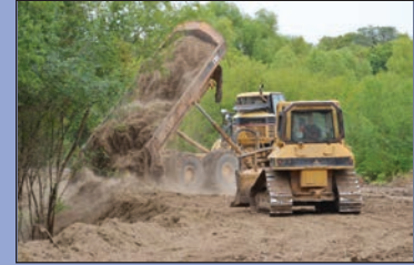
511L - Dumping material for haul road
