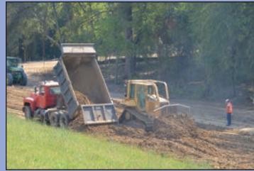
511L - Dumping material for base enlargement
