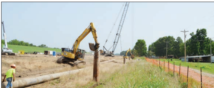
AVON - Relief Well Installation
