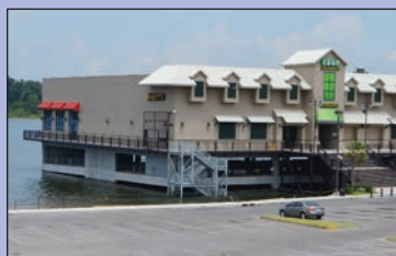
Trop Casino - lower parking area flooded
