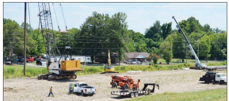
AVON - Relief Well construction
