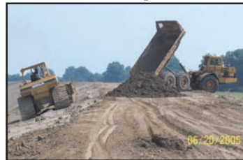
Topping out the levee
