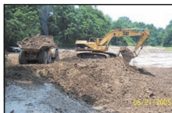
Loading dump trucks in borrow area
