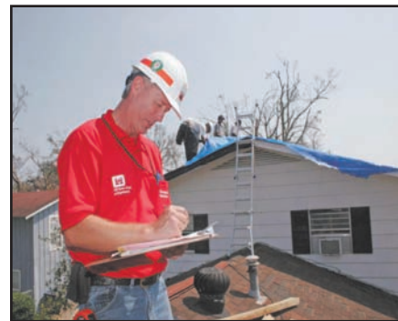
Corps employee inspects installation of Blue Roof.
