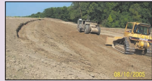
Compacting material back into levee.
