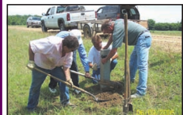
Crew installing station markers
