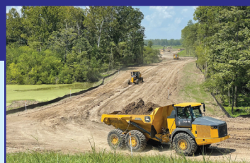
Item 452L & 458L: Loading and Hauling from Riverside Borrow Pit
