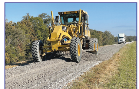
Spreading limestone on the Levee
