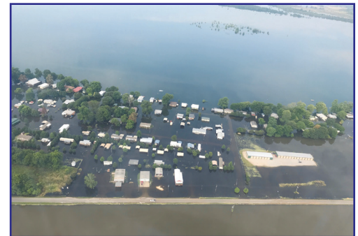
Eagle Lake Community flooded - Backwater 98.2' (May 23, 2019)
