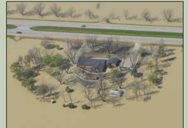
Leland - House Flooded Along Hwy 82
