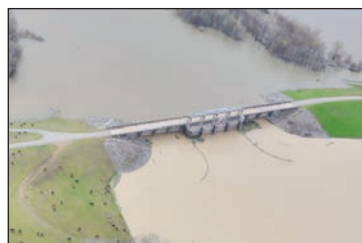
Aerial of Steele Bayou Structure
