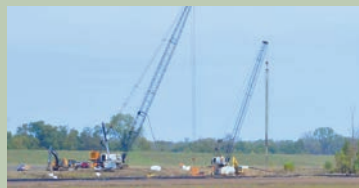
Ben Lomond Relief Well Installation
