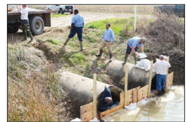
Crew Blocking Up Culverts in Valewood Ditch
