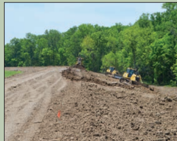
509L - Final Grading
