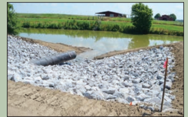
Completed Outfall Pipe
