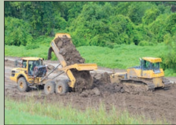
465L - Unloading Borrow Material
