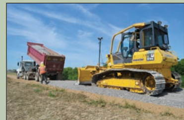
509L - New Limestone Road Surface on Completed Levee
