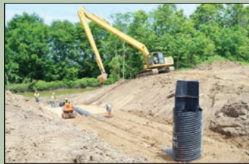
Filling in Around Outfall Pipe
