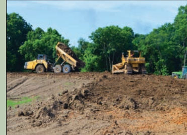
511L - Topping Out The Levee
