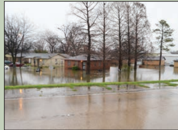
Greenville - Homes Flooded Along Broadway
