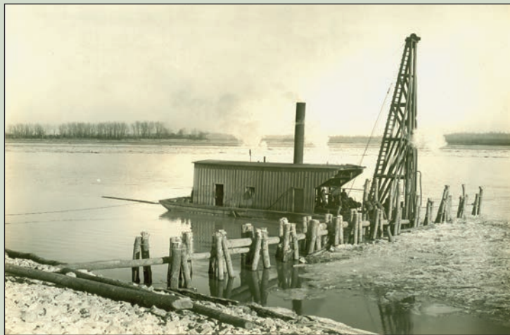
Timber Pile Dike Construction
