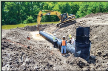
Installing Outfall Pipe
