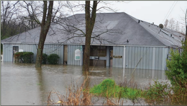
Greenville - Business Flooded
