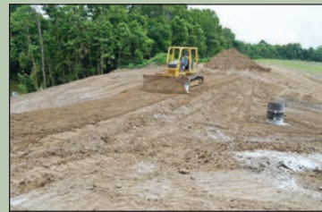
Final Grading on Levee Embankment
