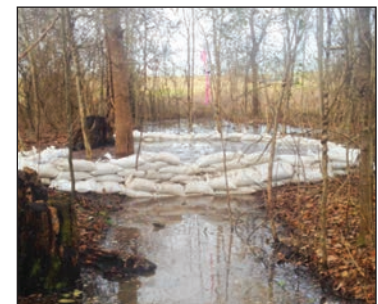
Sandbagged Sandboil at Ben Lomond
