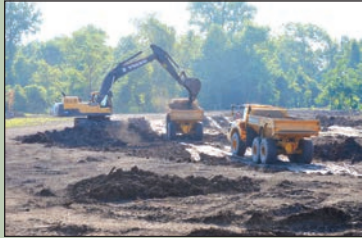
465L - Loading Borrow Material
