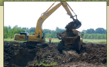
A Backhoe loads Borrow Material
