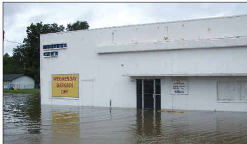
Several Businesses had considerable Flood Damage
