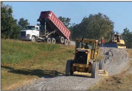
Levee Board Equipment spreading Limestone
