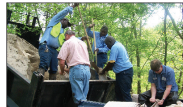
Highwater Sandbagging Operations
