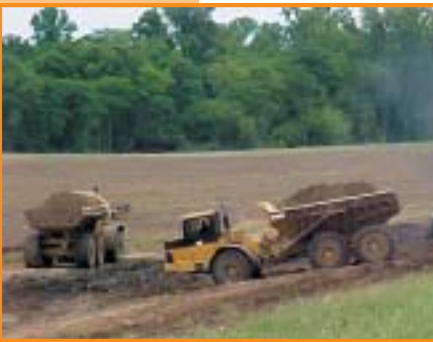
Item 496L - Enlarging Base of Levee
