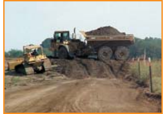
Item 496L - Topping out the Levee
