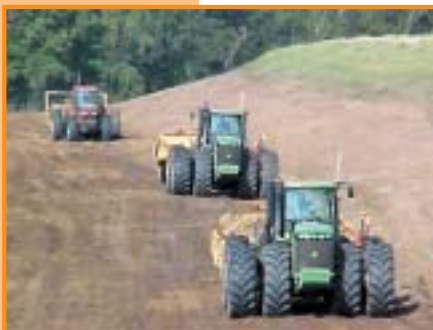
Item 477L - Enlarging Base of Levee
