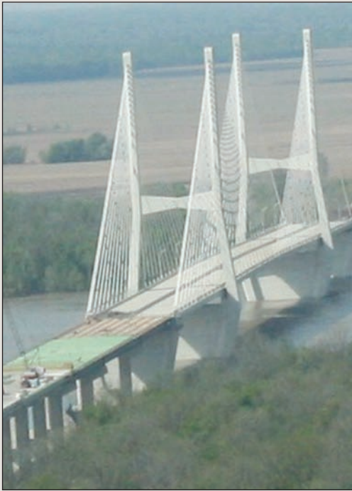
New bridge under construction.
