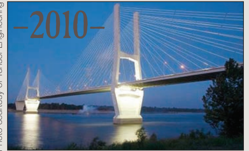
New completed Hwy 82 MS River Bridge.
