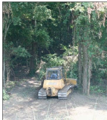
Crew clearing the 15 foot vegetation-free zone.
