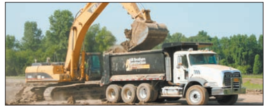
474L – Loading borrow material.
