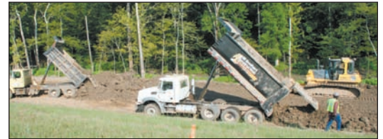
474L – Unloading borrow material.
