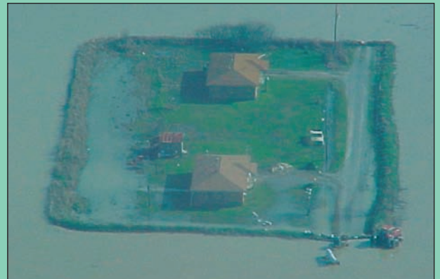
Flooding in the Darlove, MS area in December 2001.
