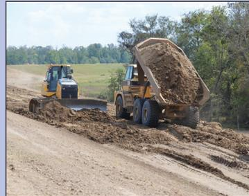
**511L - Placing and Spreading Material**
