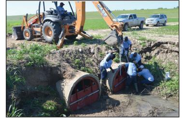
Crew Installing Culvert Weir Inserts in Valewood Ditch
