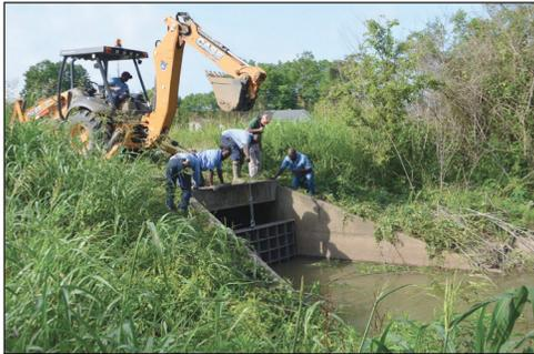
**Crew Installing Box Culvert Weir Insert at Valewood Ditch**
