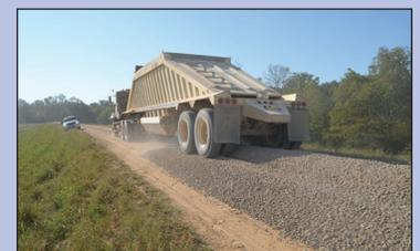
Dump Trailer Placing Crushed Stone on Levee
